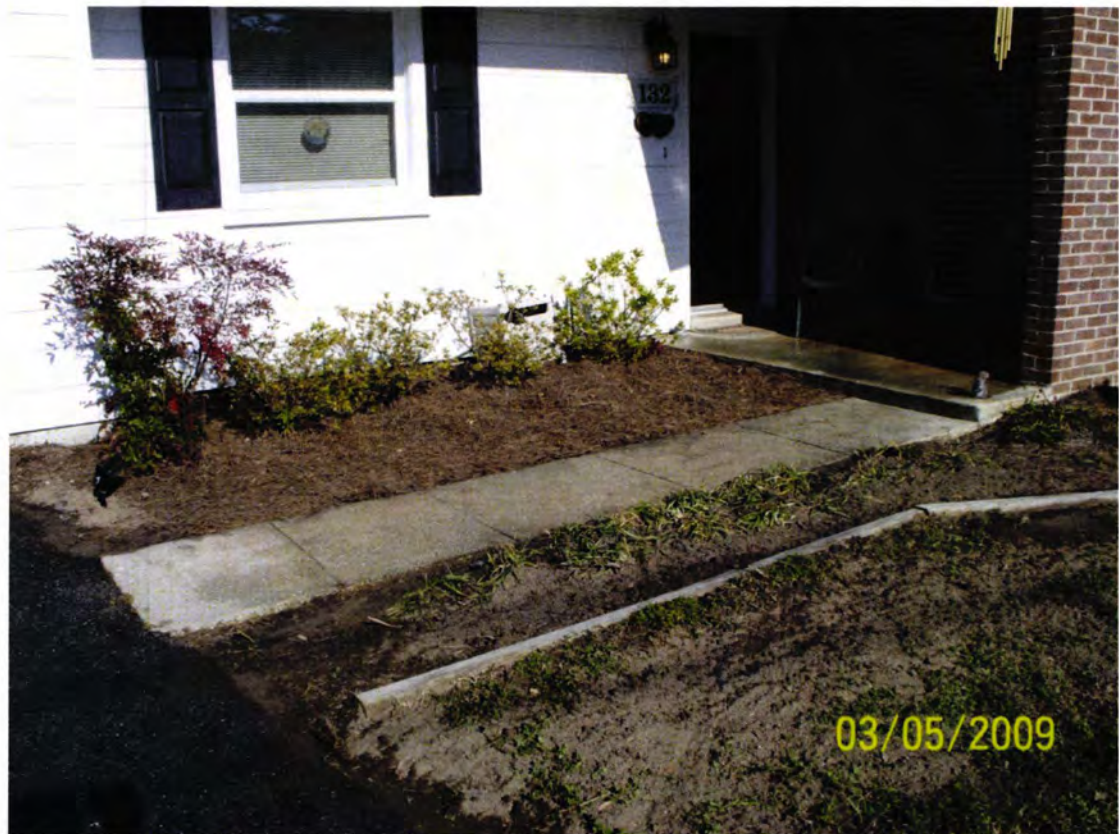
Picture 2: UST 132Banyan-1&2 after tank removals and restoration.
