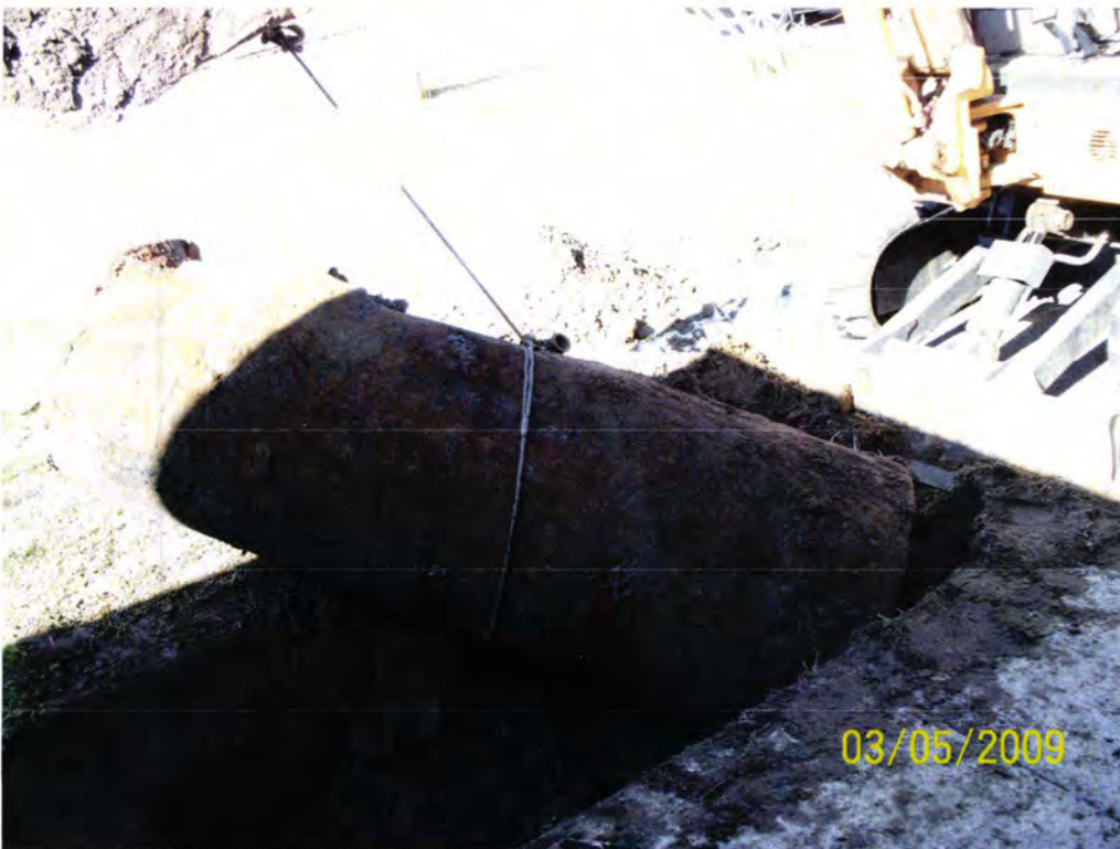
Picture 4: UST 132Banyan-2 during removal.
